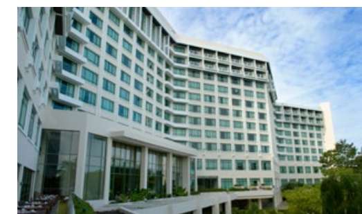
America – Office Building
